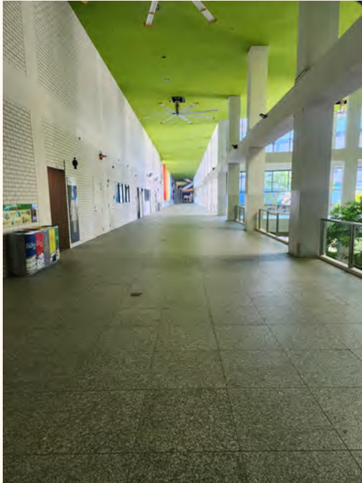
Outside TCC Level 3 Corridor (ENGINE between Block 32 & 22)
